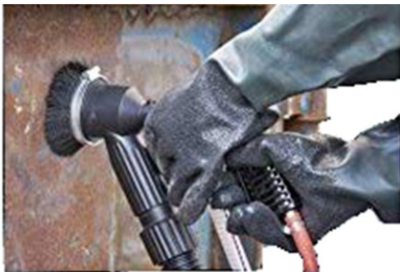
Fig. 9: Application of the blasting pistol
